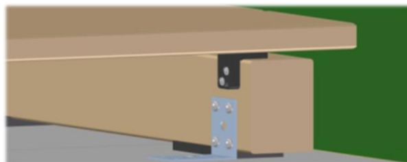
Figure 8: Screw the end clip to the substructure.
